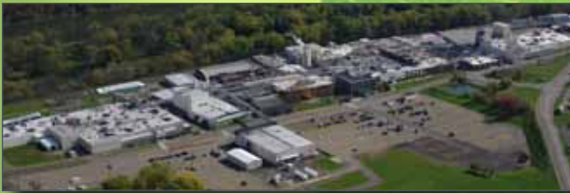
GTP Headquarters - Towanda, PA, USA Chemical Recycling
